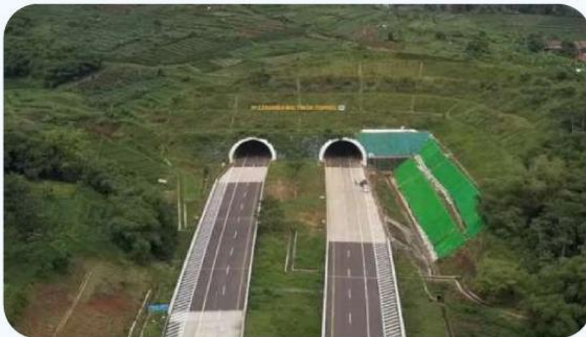
Gambar 3 : Twin Tunnel Tol Cisumdawu
