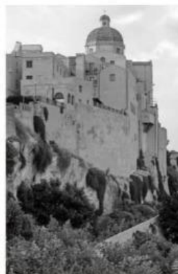
▲ Cagliari Cathedral was first built in the 13 th century and overlooks the city.
