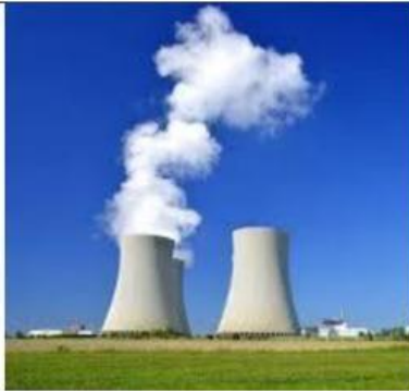
Nuclear Power Plant
