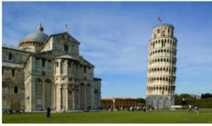
Leaning Tower of Pisa
