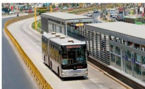
BUS STATION / BANK
