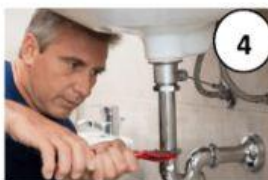
I repair water pipes.
