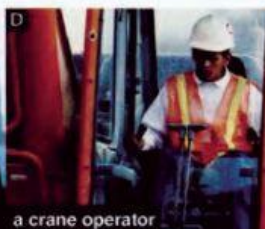
a crane operator
