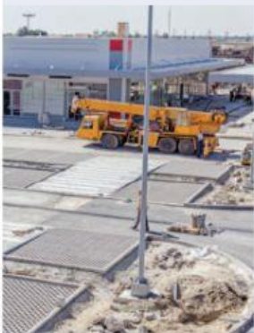
Building a new supermarket
