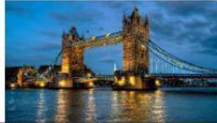
London Bridge (262 m)
