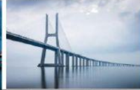
Danyang-Kunshan Grand Bridge (164.851 m)
