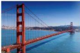
Golden Gate Bridge
