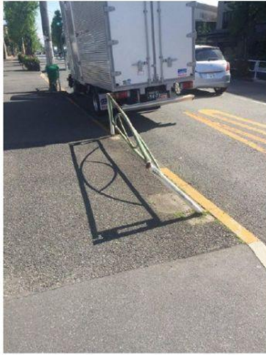
A bent gate
