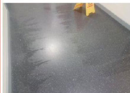
Drying of a moped floor
