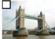
m- Tower Bridge
