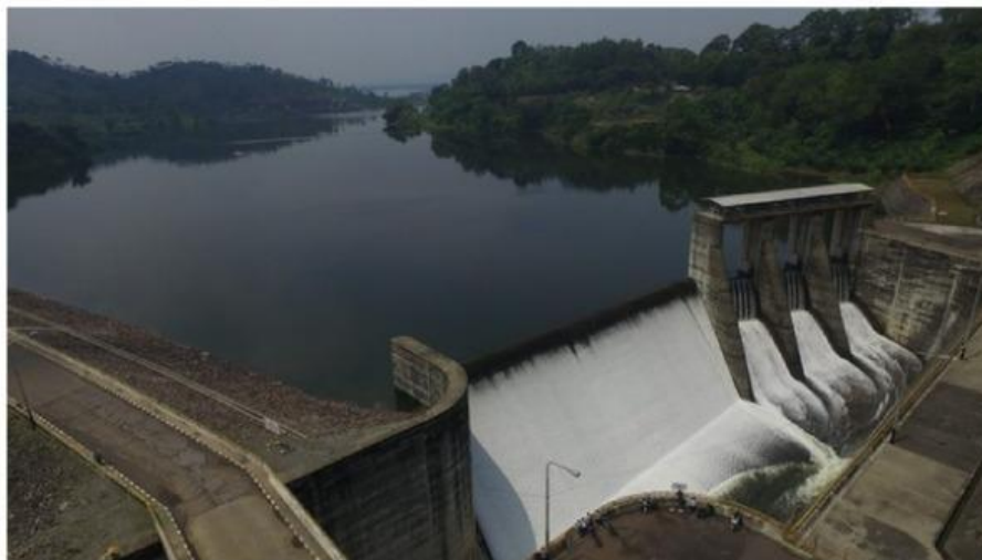
Fig 1. Saguling Hydroelectric Power Plant
