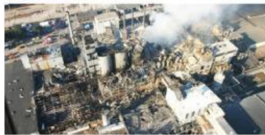
Gambar 2. Kerusakan Pabrik Imperial Sugar Pasca-Ledakan Debu Gula
