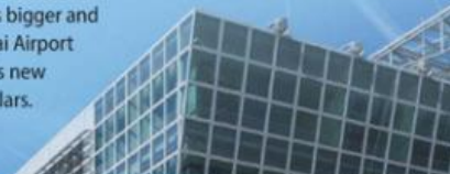
Munich International Airport
