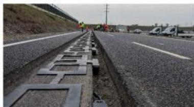
This technology can be useful for buses, trucks, and taxis that drive all day. It saves time and reduces the need for big batteries. According to Electreon, 1 km of wireless road can charge a car enough for 20–30 km of driving.
