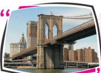
This bridge built between 1869 and 1883 by an engineer John Roebling. It is world's first steel wire suspension bridge. It has a main span of 1596 ft.
