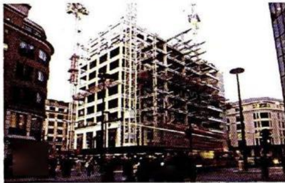
Steel beams make taller structures possible.
