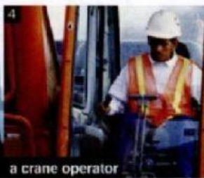
a crane operator
