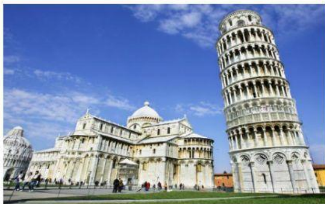
Leaning Tower of Pisa
