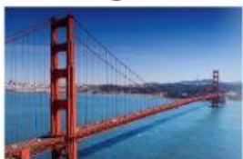
Golden Gate Bridge
