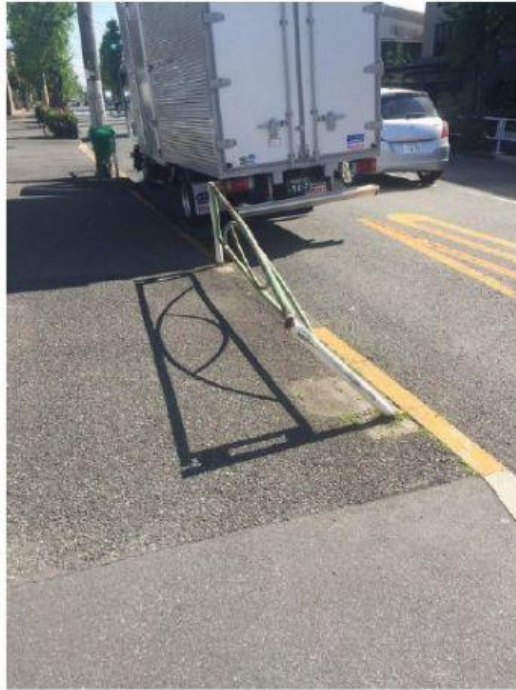
A bent gate
