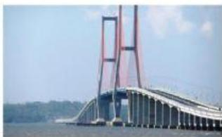
The Suramadu Bridge is also known as the Surabaya-Madura Bridge with three cable-stayed sections constructed between Surabaya and in the island of Java to Bangkalan in the island of Madura in Indonesia.
