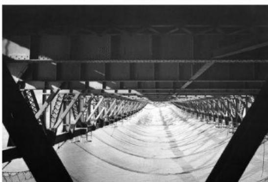
During construction, a safety net was suspended under the floor of the bridge, extending 10 feet wider than the bridge's \_\_\_\_\_ and 15 feet longer than its length. The net proved an invaluable precaution as it saved the lives of 19 men. These men became known as members of
