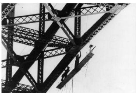
In the 1930s, the Golden Gate Bridge was coated with a primer that was two-thirds (by weight) lead. The architects intended the lead-based paint to protect the steel structure from corrosion, but later learned that lead is harmful to humans and the environment.
