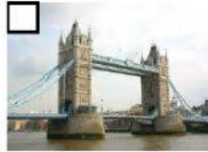
m- Tower Bridge
