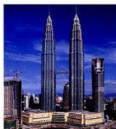
Petronas Twin Towers
