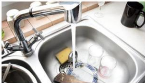
The faucet with running water
