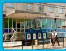
3 a police station
