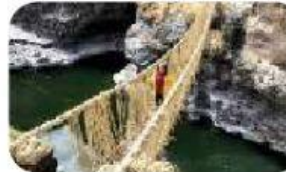
Q'eswachaka Inca Bridge
