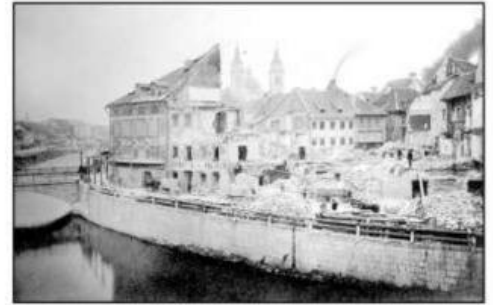
April 14, 1895, a big earthquake hit Ljubljana. The earthquake damaged buildings throughout the city. 7 to 12 people died.
