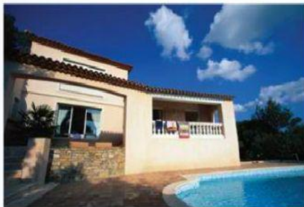
A flat/apartment with swimming pool
