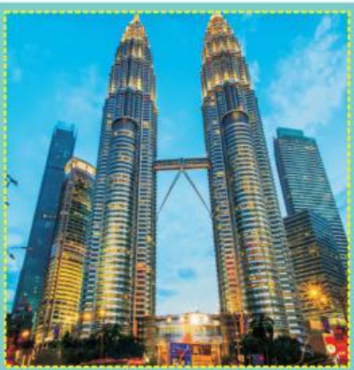
Petronas Twins Towers (1,483 ft)
