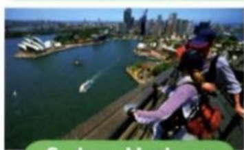
Sydney Harbour Bridge
