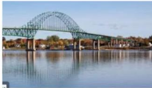
The Centennial Bridge over the Miramichi
