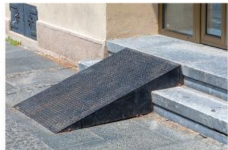
An inclined plane used as a ramp at the wheelchair and trolley entry at the front of the building
