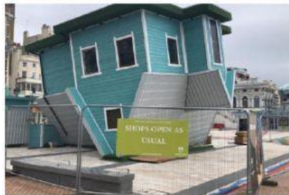
upside- down house
