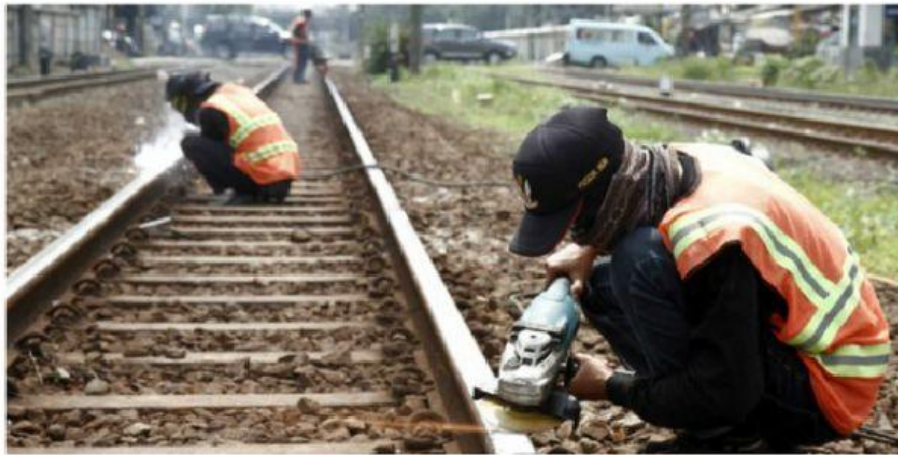
Perawatan rel kereta di Cipinang. ©2016 merdeka.com/muhammad luthfi rahman
