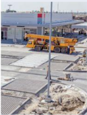
Building a new supermarket
