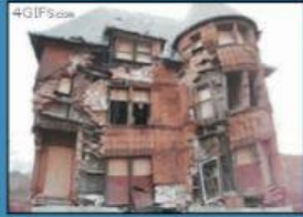
The house collapsed .
