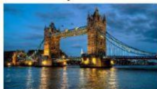
London Bridge (262 m)
