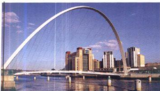
Gateshead Millennium Bridge
