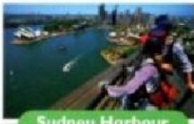
Sydney Harbour Bridge
