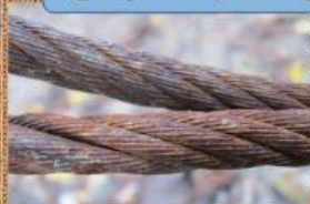
rusting of cables
