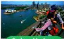
Sydney Harbour Bridge
