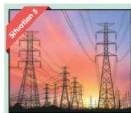
The electric cables are hung loosely between the electric poles to allow the wires to \_\_\_\_\_ when the temperature decreases.
