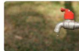
water droplets from leaky faucet
