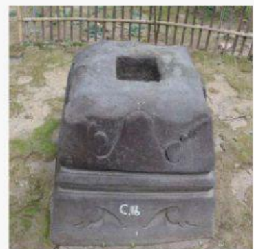
Gambar 4. Umpak Pendopo
